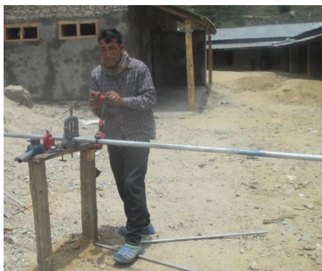
Nanda Ram Rokaya fitting the water pipe
